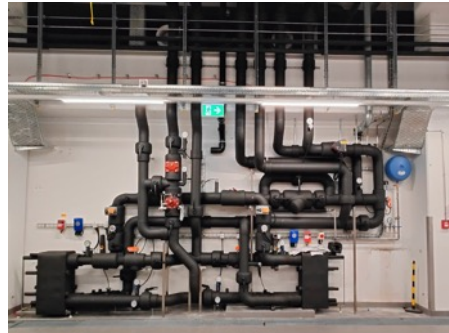
Underground water exchangers
