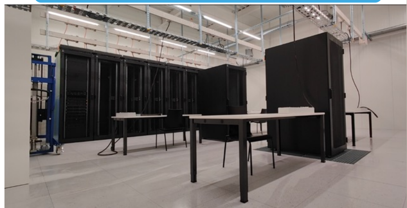
Racks with air/water passive cooling
