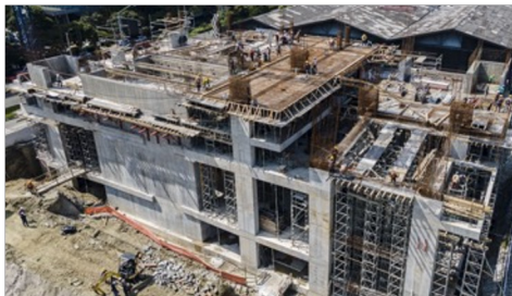
Building in construction, Columbia © Argos Cements
