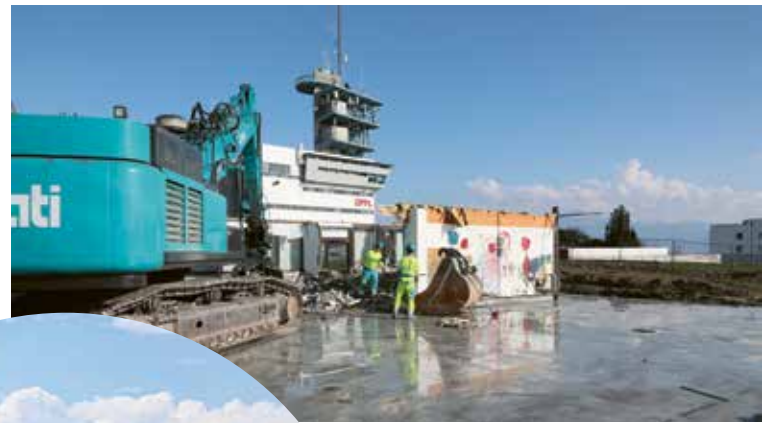
Construction site of the RTS building.
