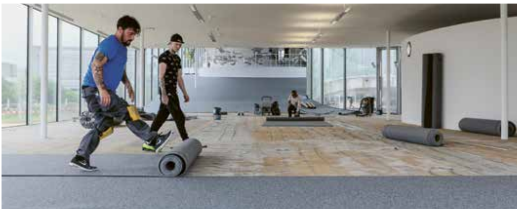
Laying of new carpet at the Rolex Learning Center.
