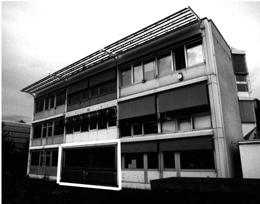
Figure 3.1 : South facade of the LESO building (the rooms used for the DELTA experiment are highlighted with a thick line)
