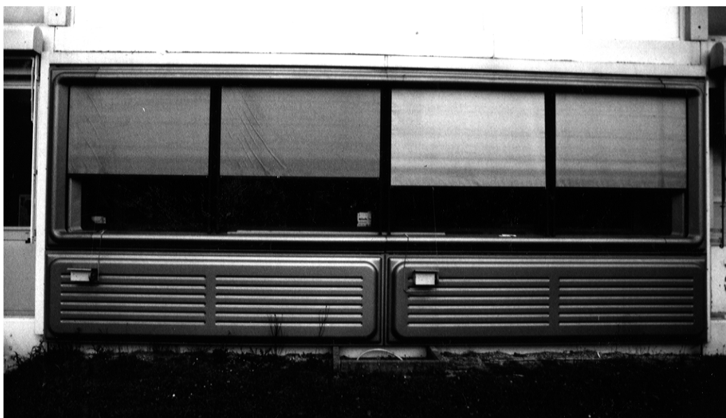
Figure 3.2 : A closer view of the test rooms' facade
