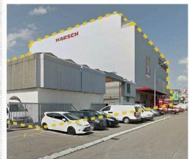
date of construction : 1972 address : rue Baylon 10, Carouge typology : storage building
