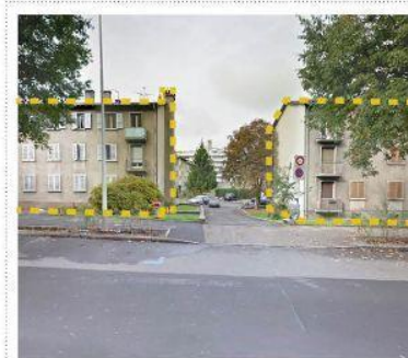
date of construction : unknown address : rue de la Fontenette 33, Carouge typology : residential building
