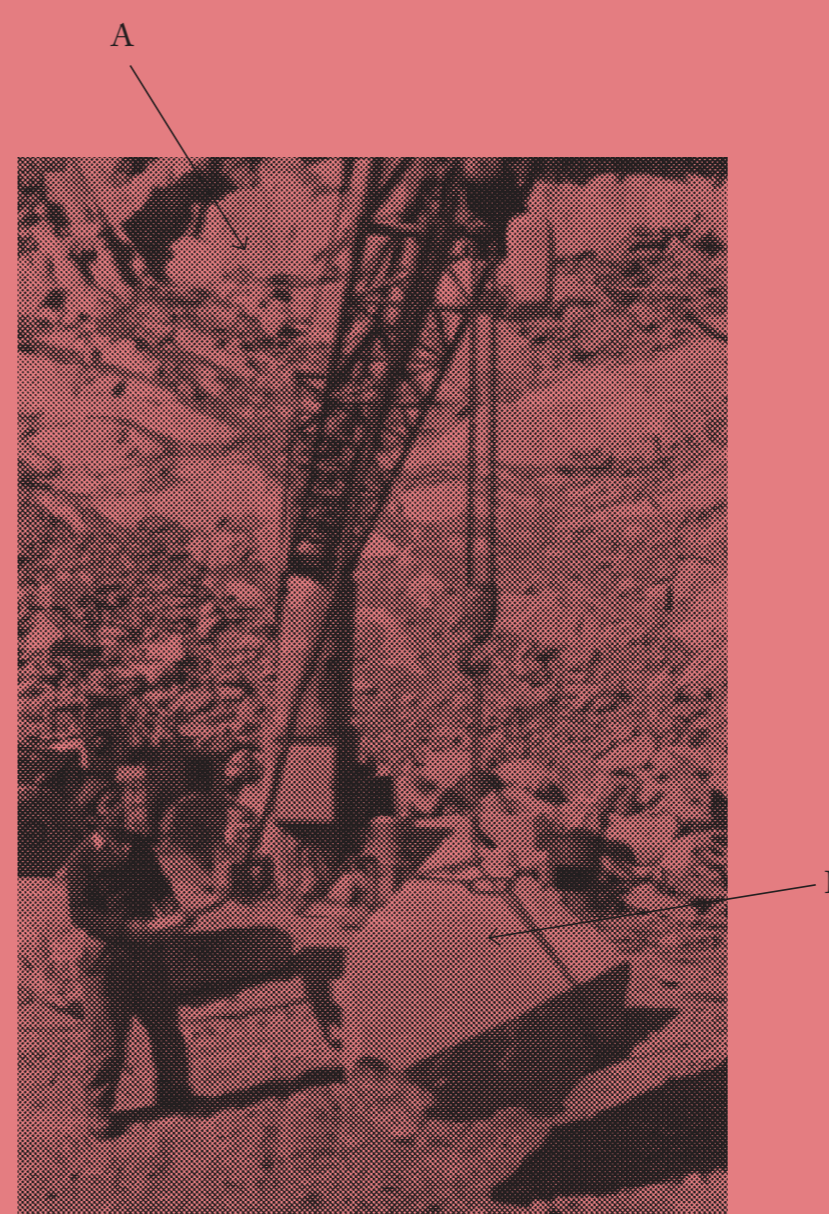
[A] Andeer, granite quarry, 1976. Schmid, Walter. ETH Library Zurich
