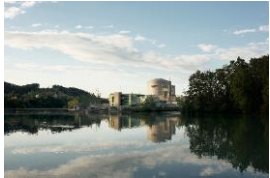
NPP Beznau I & II (KKB I / II) PWR, 2x 365 MWe Westinghouse 2 Loop Sept. 1969 / Dez. 1971
