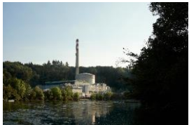
NPP Mühleberg (KKM) BWR, 373 MWe GE BWR 4 / Mark 1 Nov. 1971 – Dez. 2019 (in decommissioning)
